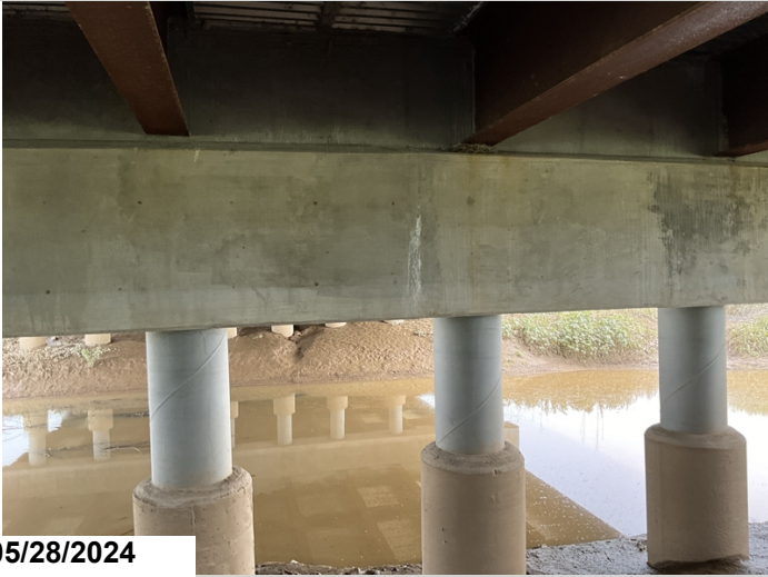
Bent 2 & 3, Pile Cap, Both Sides, At Construction Joint: Hairline crack with light efflorescence. 2LF CS2 (Efflorescence/Rust Staining)
