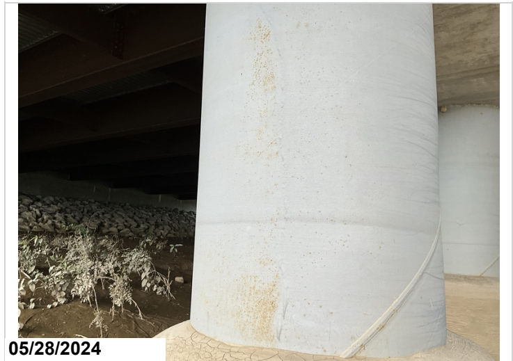
Bent 2 & 3, Steel Piles, About Concrete Encasement: Areas of surface rust. 725SF CS2 (Effectiveness)
