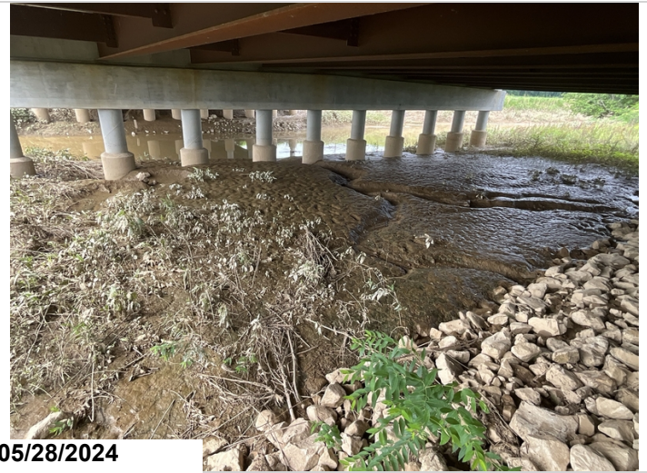
Span 3, Channel Slope: Few minor erosion veins running down slope.
