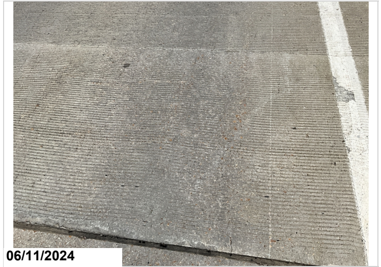
All Spans, Deck Surface, Full Length: Areas of CS2 cracks. 1510SF CS2 (Cracking)
