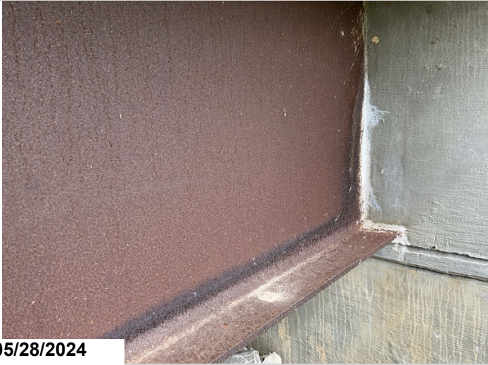
Span 3, Steel Girder, At Bent 4, Right Side: Active corrosion with light laminations for 1'.
