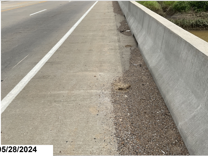
All Spans, Deck Surface Gutters: Dirt and debris.
