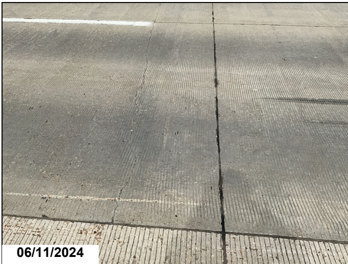
Abutment 1 & 2, Approach Slab: Cracks. 250SF CS2 (Cracking)
