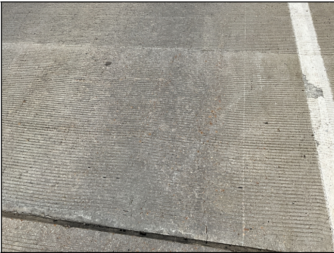
All Spans, Deck Surface, Full Length: Areas of CS2 cracks. 1510SF CS2 (Cracking)
