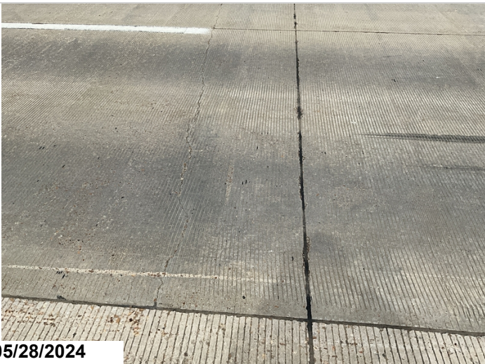
Abutment 1 & 2, Approach Slab: Cracks. 250SF CS2 (Cracking)
