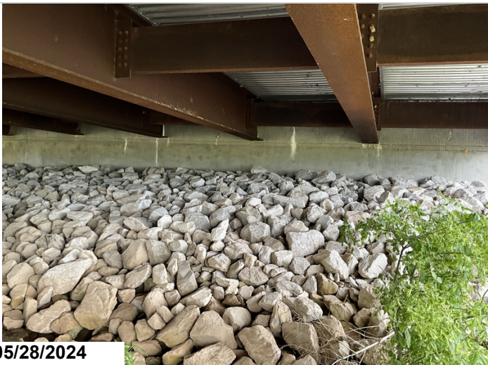
Abutment 1 & 2, Back Walls: Hairline vertical cracks some with light efflorescence. 23LF CS2 (Efflorescence/Rust Staining)
