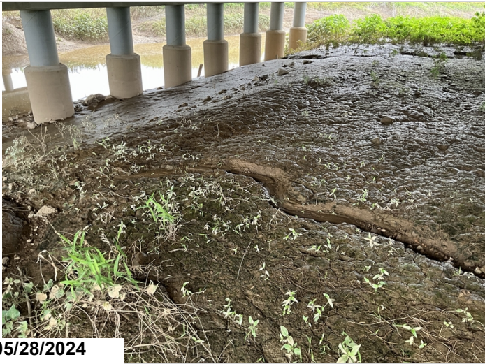
Span 1, Channel Slope: Few minor erosion veins running down slope.
